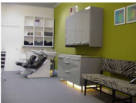
Decorative mortar in a barber shop (Primer 300 gr/m 2 , 13 kg UniQuartz TK 11 with binder 12% of the filler, Topcoat 200 gr/ m 2 EP Thix 300)
